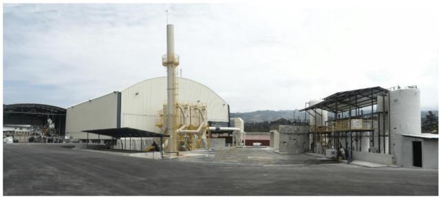
Pb Metals 2012: L to R - used batter breaker - smelter and refinery - baghouse - ETP
